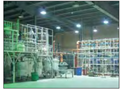
The new DMCC-accredited gold refinery was opened in 2004.
