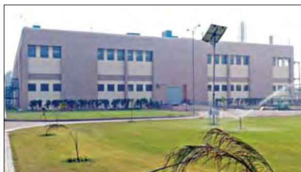
The refinery's 10-acre site is so large that a vegetable garden provides fresh produce for the staff canteen.
