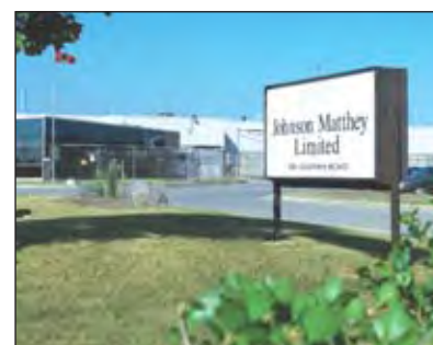
The plant at Brampton near Toronto airport manufactured minted bars from 1990 until 2000.
