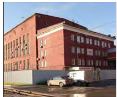
The headquarters of Uralelectromed has been located in Lenin Street in Verkhnyaya Pyshma since 1978.
