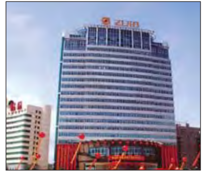
The international headquarters of Zijin Mining in Shanghai.
